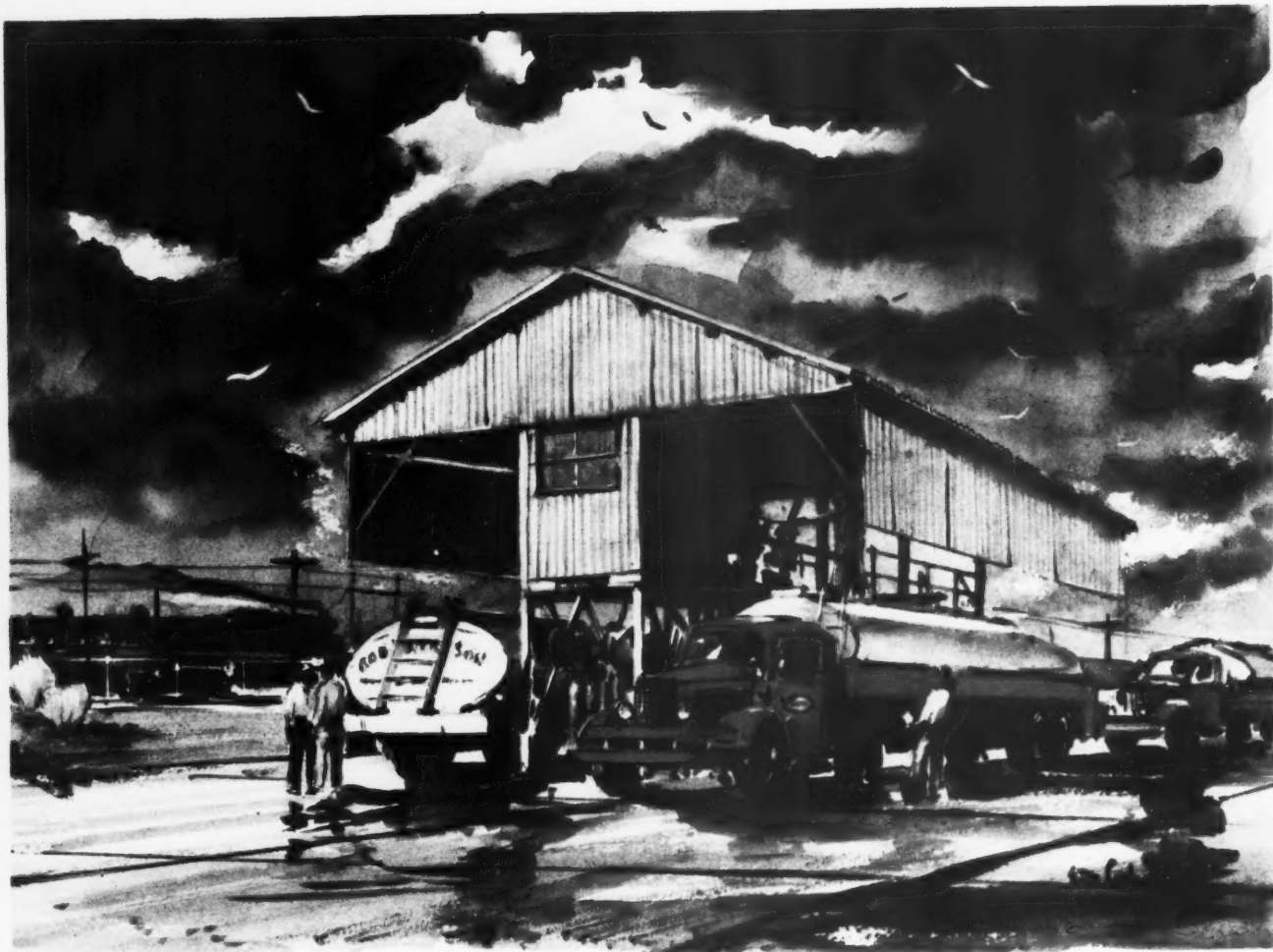
Busy Gasoline Terminal
